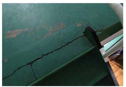
Photograph 3: Floor slab cracking at top of stairs.
