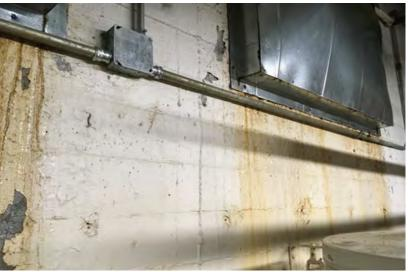
Photograph 1: Water infiltration at existing wall openings that have been infilled.
