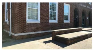
**GYM RAMP** SLOPE OF RAMP RANGES FROM 7.6% TO 9.6%. A HANDRAIL IS NEEDED TO MEET CODE
