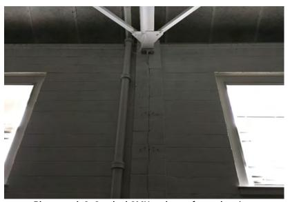
Photograph 2: Cracked CMU under roof truss bearing.
