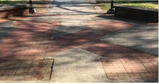
1 CENTER OF QUAD BRICK INLAY IS SETTLING AND NEEDS TO BE REMOVED AND REPLACED WITH PROPER SUBBASE.
