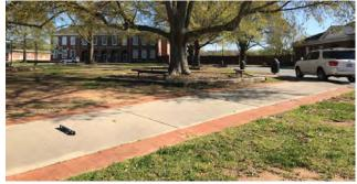
SIDEWALK CROSS SLOPE CROSS SLOPE OF EXISTING SIDEWALK DOES NOT MEET CODE
