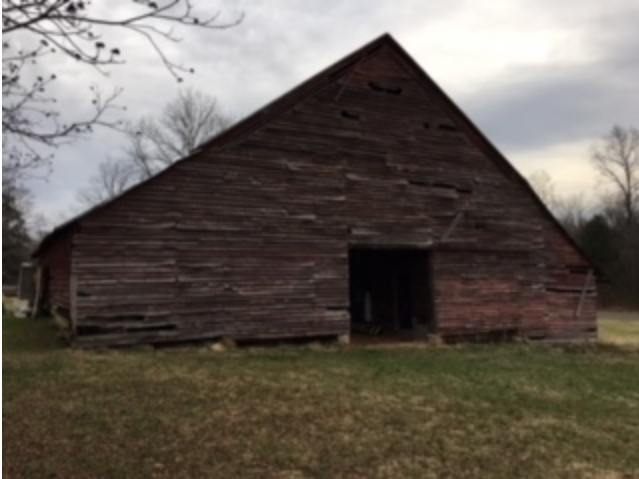
Barn view from the South
