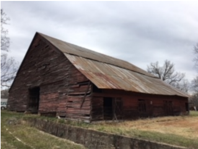
Barn view from the South East
