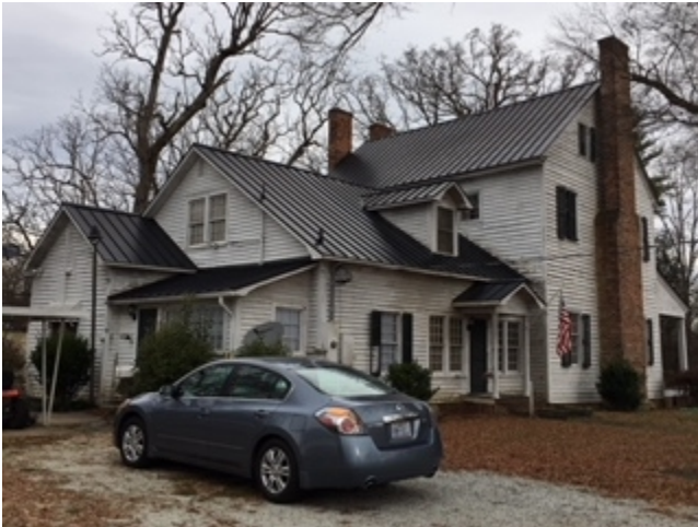
House view from the south.
