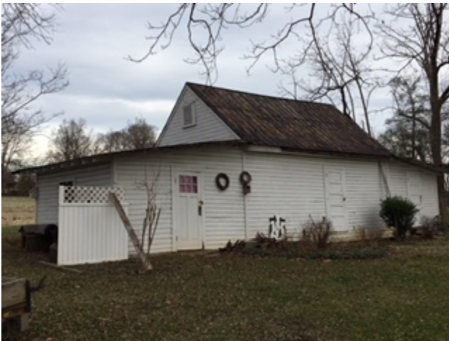
Smoke house view from the North
